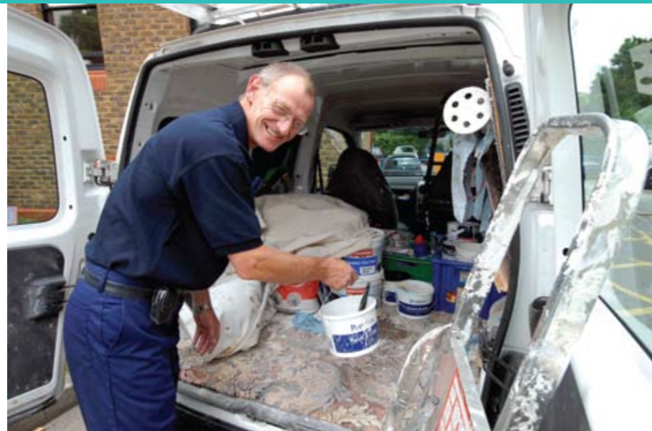
A KBS workman about to carry out some work on a ‘void’ property.
